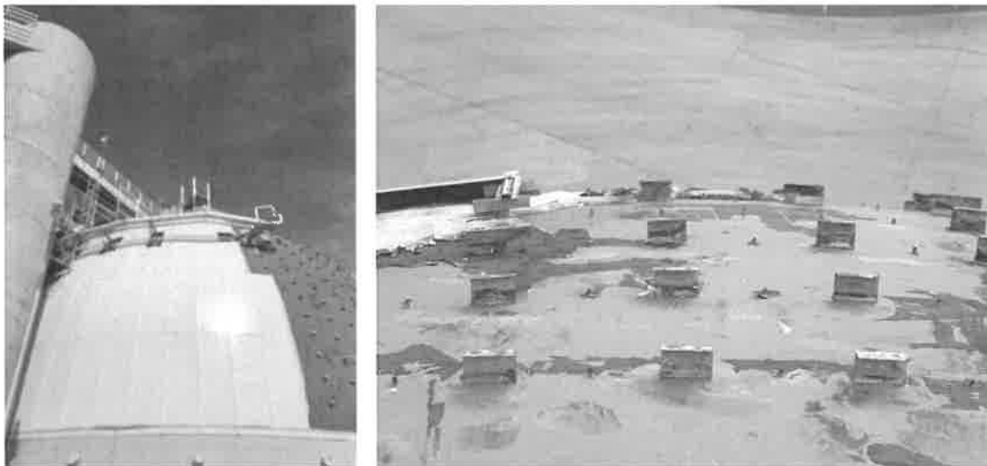
Figure No. 3: Corroded Digester Plate Discovered During Construction
