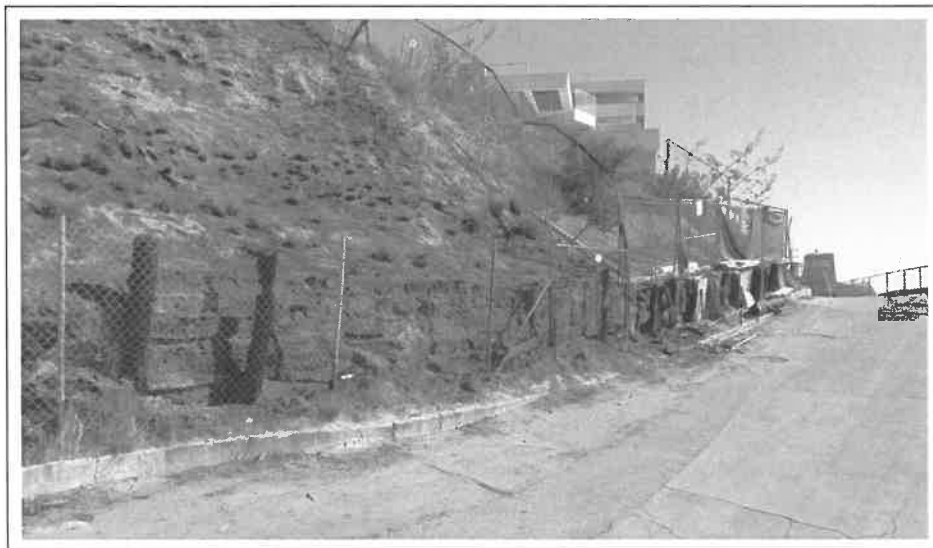
Figure No. 1: Castellammare Drive fire damaged timber bulkhead
