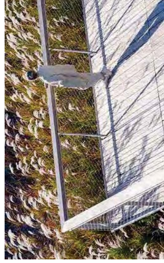
Bi-directional bikeway with gabion retaining walls to hold slope and planting area
