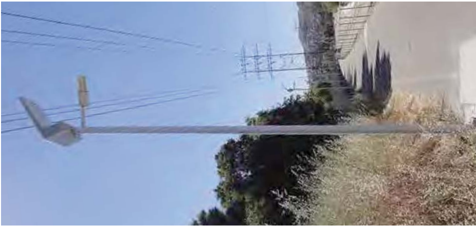
Hybrid solar lighting on existing LA River bikepath
