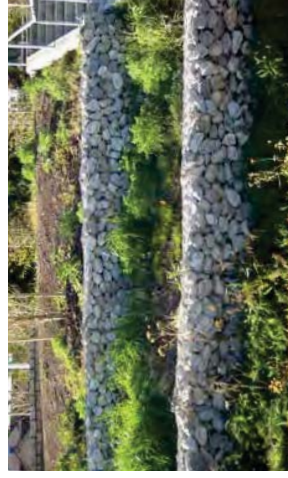
Gabion walls to retain existing slope planting
