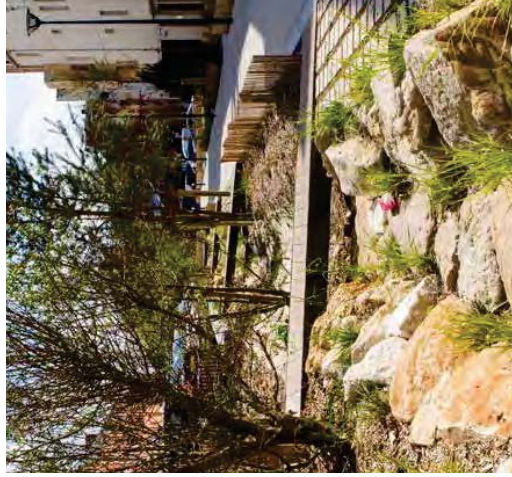
Street end bioswale will filter and infiltrate stormwater before entering the LA river
