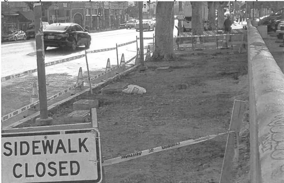
String line set-up for ADA compliant sidewalk slope, ready for Urban Forestry root-prune.
