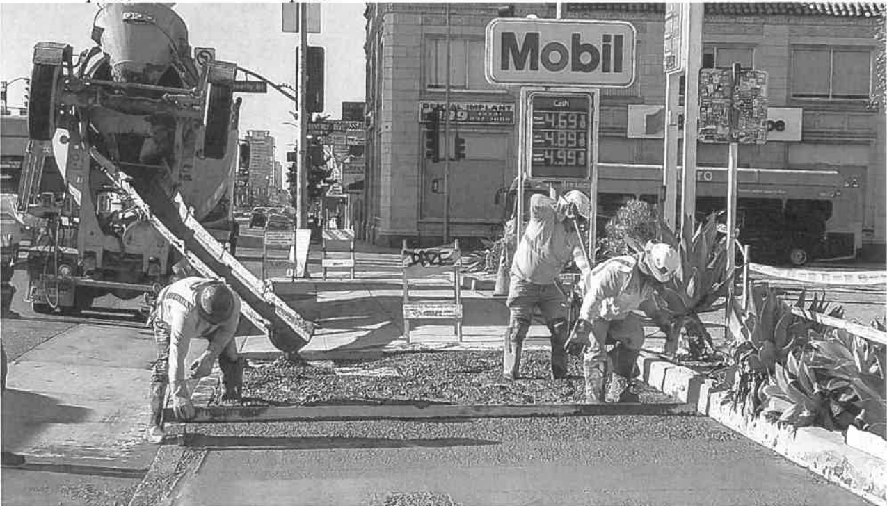
Concrete pour, and initial finish pass.
