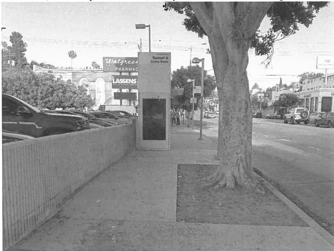
Installed shelter, ADA compliant sidewalk, root uplift corrected - view looking east
