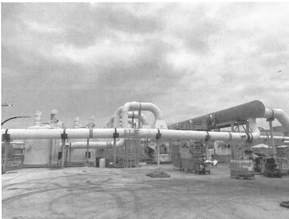
Figure: Existing Chemical Scrubbers at Primary Batteries
