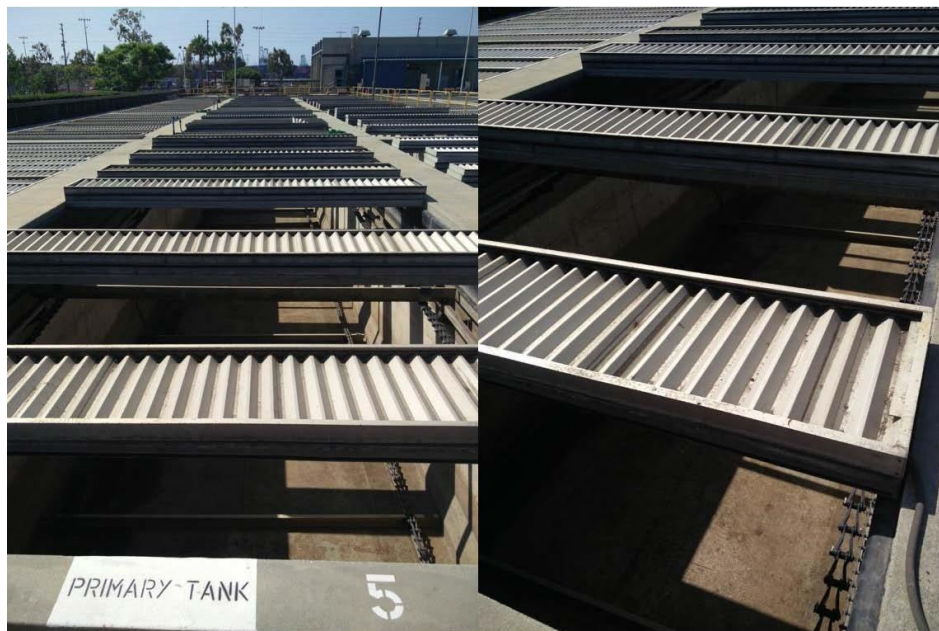
Figure No. 2 - Covers at primary sedimentation tanks at the TIWRP.
