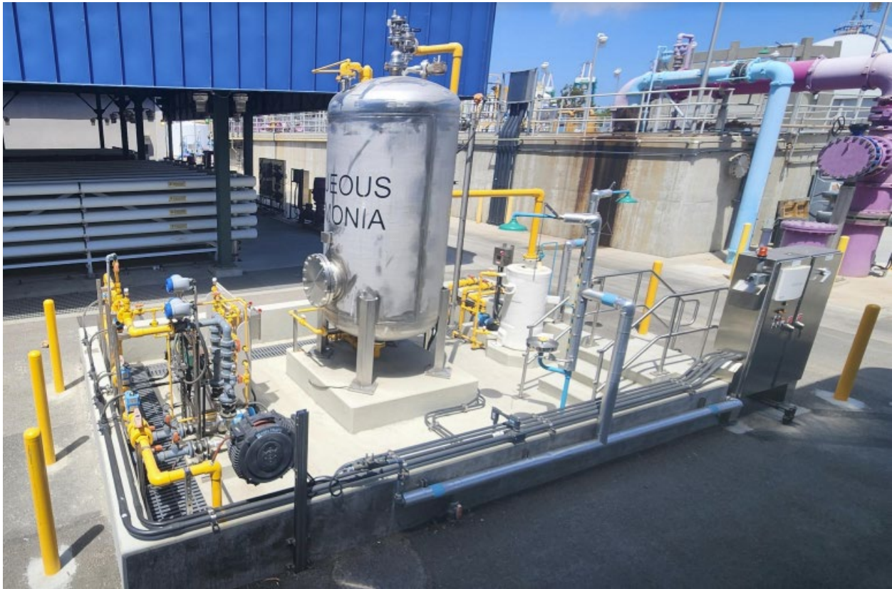
Figure No. 1: Ammonia Injection System completed under CIP 5125 Terminal Island Wastewater Reclamation Plant Advanced Water Purification Facility Advanced Oxidation Process Ammonia Injection System
